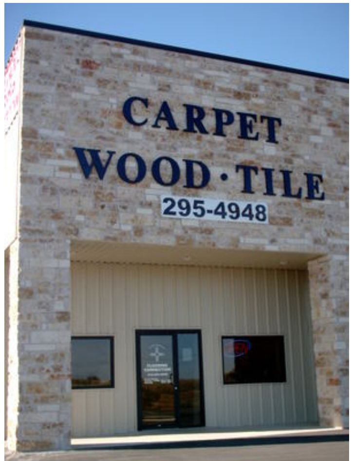
View of End of Building
