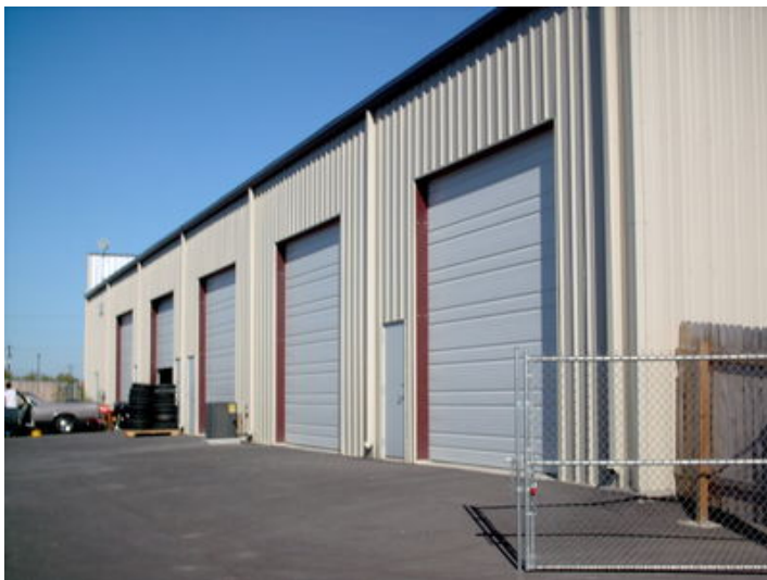
View of Rear of Building
